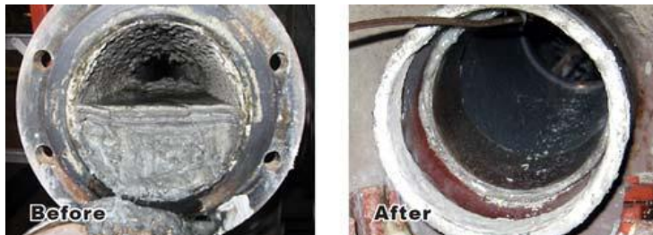
Existing Stage 2 Eductor Headers were extremely fouled with oily sludge resulting in very poor flow and distribution of pumped process solution.
