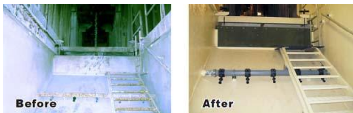
Stage 4 Steel stairs, handrails, and internal piping were extremely corroded.
