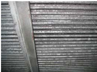
Reheater tubes detailing corrosion
