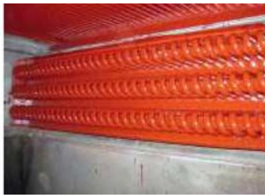
Tubes abrasive blasted and primed with Red ChemLINE 784-32
