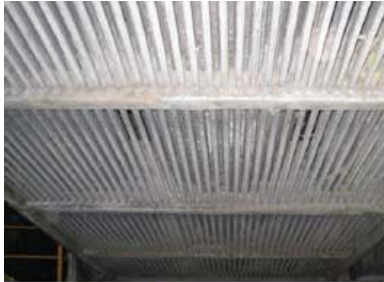
Reheater tubes before lining.
