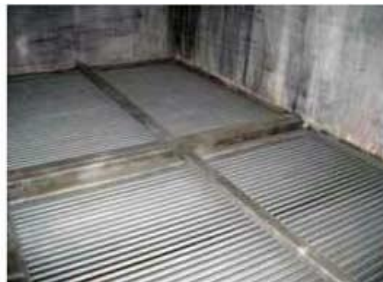
Reheater tubes viewed from above after blasting and before lining
