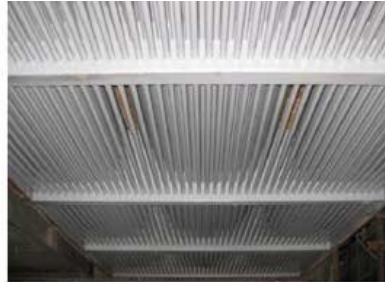
Reheater tubes after lining.
